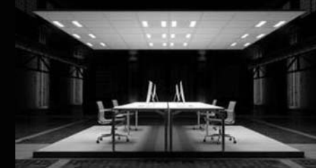
After, with Linessa Air and integrated ventilation.
